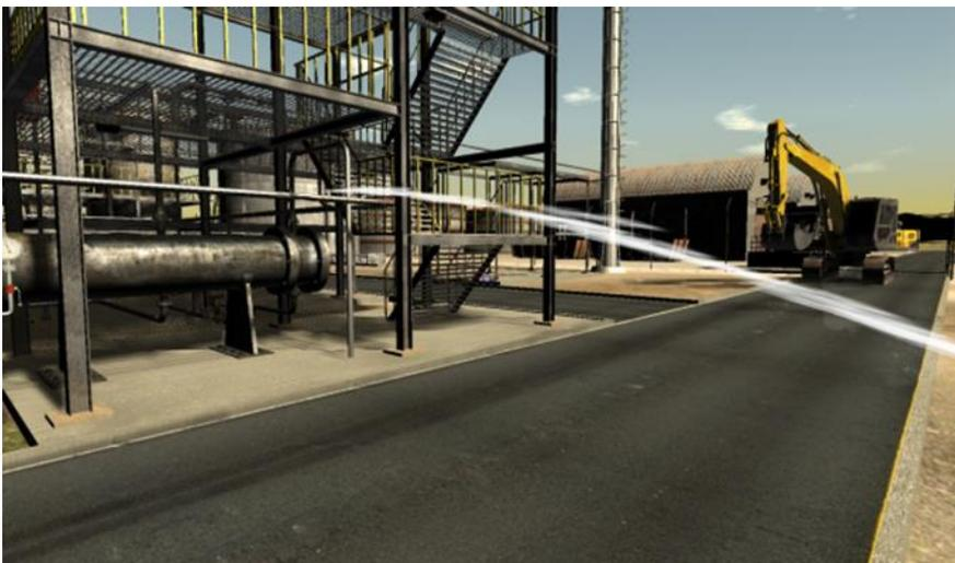
*Figure 1. Liquid leakage from the ruptured flange (courtesy of Virthualis Srl).*
